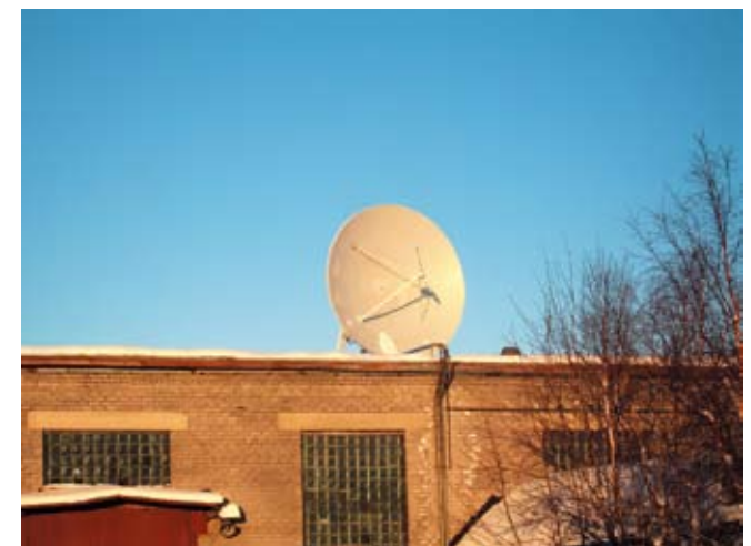
Satellite antenna of Rosatom communication system
