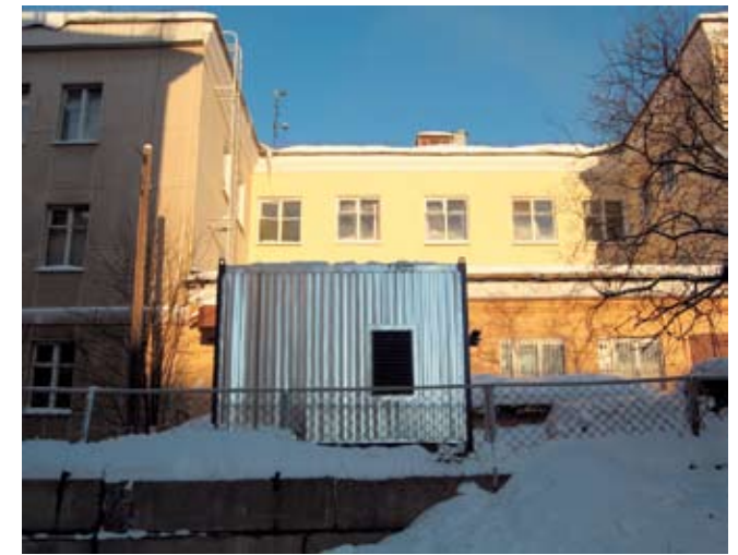
Diesel Generator Container
