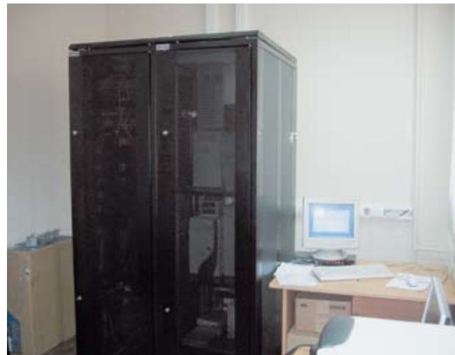
Server and communication equipment of Murmansk ARMS
